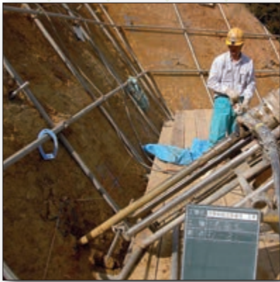
切土補強土工
