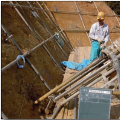
切土補強土工
